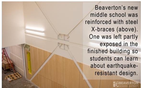
Beaverton's new middle school was reinforced with steel X-braces (above). One was left partly exposed in the finished building so students can learn about earthquake-resistant design.
