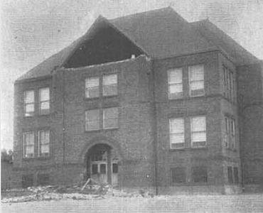
Above: Lafayette Elementary School in West Seattle was condemned and torn down due to damage from a M7.1 earthquake in 1949.
