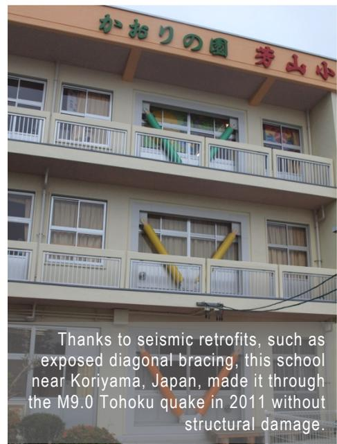
Thanks to seismic retrofits, such as exposed diagonal bracing, this school near Koriyama, Japan, made it through the M9.0 Tohoku quake in 2011 without structural damage.
